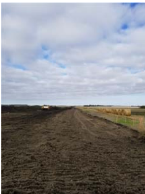
Back fill at Shoe Fly 5, Photo taken facing west
