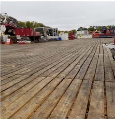
Good housekeeping at HDD site Dead Horse Creek
