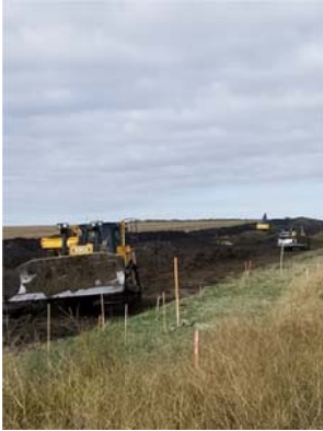
Back fill crew working at Shoe-Fly 7 Photo taken facing West
