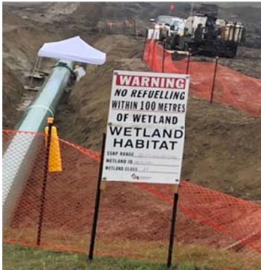
Completed road bore at SSKP 1015
