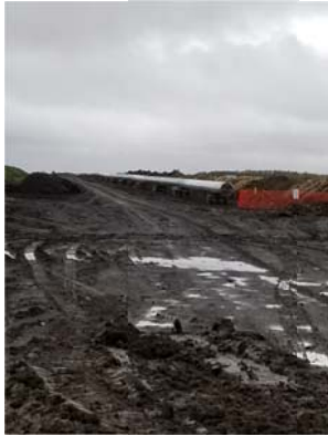
ROW access at Shoe-Fly 17 Photo taken facing East
