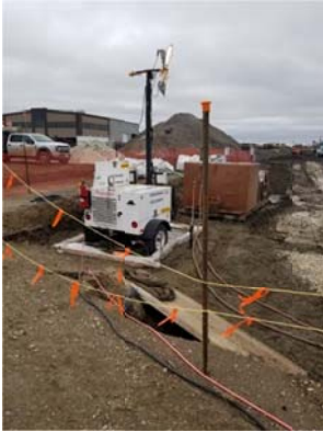
Environment precautions at Road Bore South of Highway 3. Drip tray underneath light Plant. Photo taken southeast.
