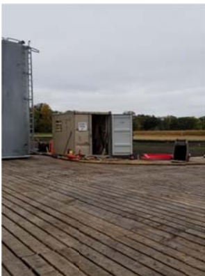
Environment response trailer at Dead Horse Creek HDD site, photo facing northeast.
